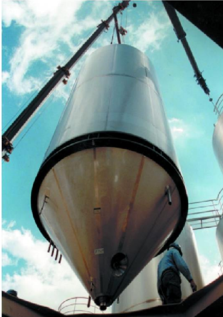
■ Figure 1. Installation of a batch, 765-bbl beer fermenter made of stainless steel. (Courtesy of Paul Mueller Co.)
