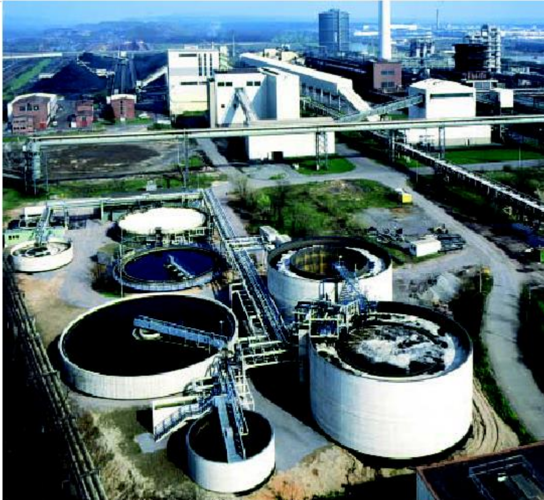
Wastewater Treatment Plant for a coke oven complex at Dillingen /Germany (LINDOX® and LINPOR®-N)
