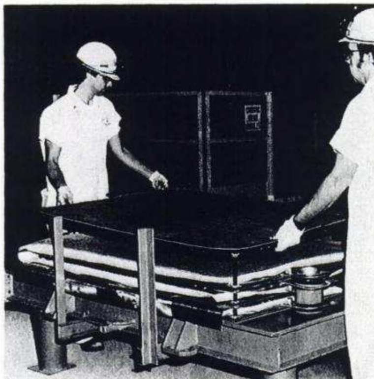
Fig. 3.14 The construction of an MGC electrolyser. (Courtesy: OxyTech Systems Inc.)
